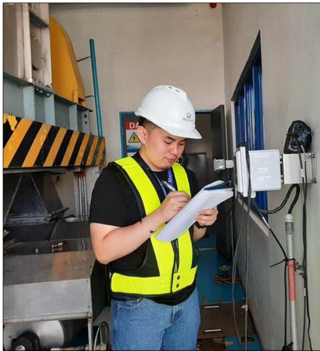
Picture 1. Recording the results of pH and DO of Aerated Water in Alabang-Zapote Septage Treatment Plant
